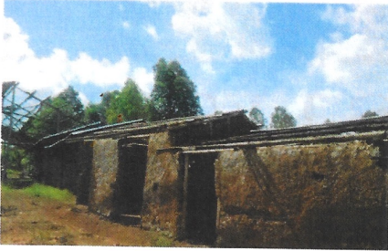
Old School Building
