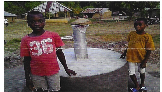
Sierra Leone rural village well water pump Almost complete
