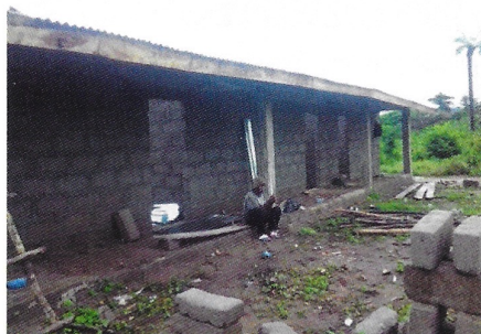
Orphanage school being roofed.
