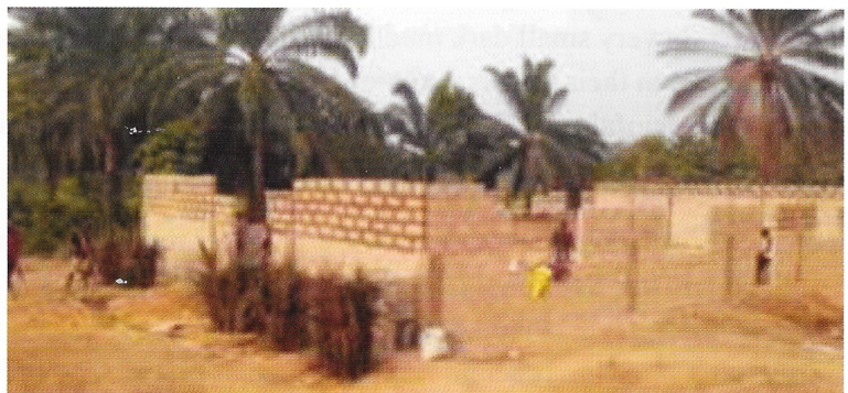
School & Church building under construction
