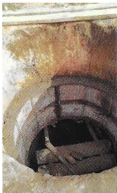
Almost complete well In Sierra Leone
